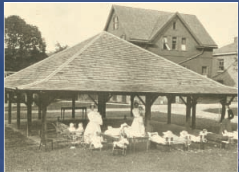
Harmony Circle Pavilion, West Genesee St., 1903.
