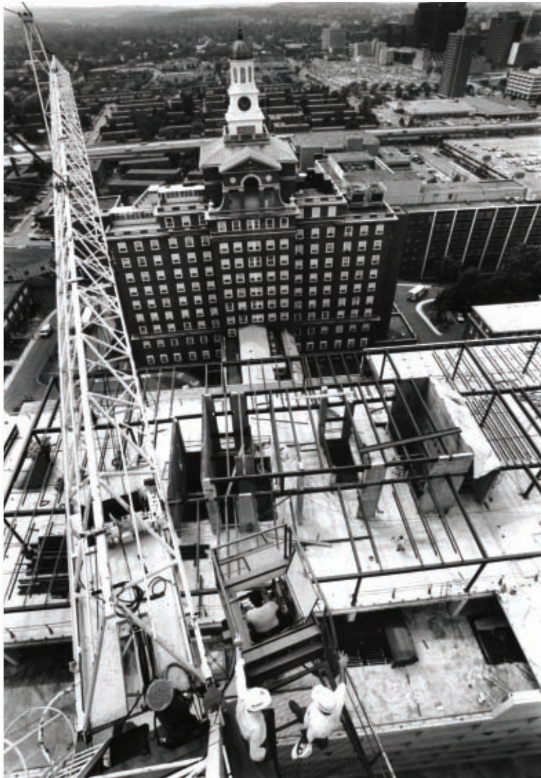
Construction of Irving Unit, 1973.
